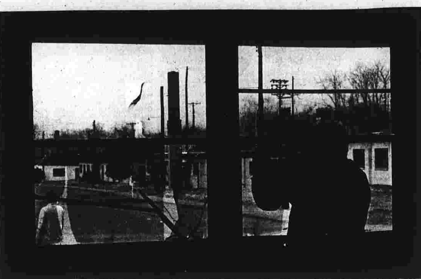
In all of the many windows of the buildings, slashed screens, like this one had to be completely cut out and the rest of the glass in broken windows had to be removed.
